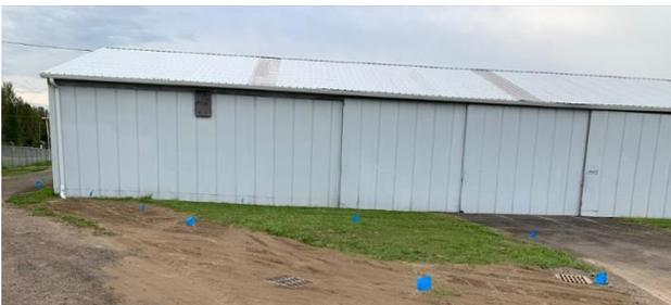
You'll notice that several new drain boxes have been installed on the south side of the hangars along the taxiway and that our gutter drain lines now connect to the airport drainage system.
