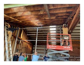
On another weekend, Dan painted the frames. Then came the moment of truth: remove one old door and hang a new door frame. The guys took down the old door gingerly and without incident. Likewise, we manually lifted the new door frame into place. The door frame fit like a glove and rolled smoothly on refurbished wheels.
