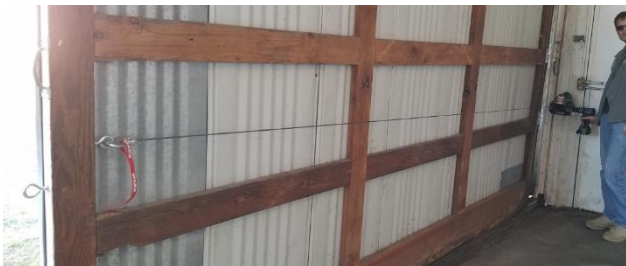
Using the winch to pull the door open
